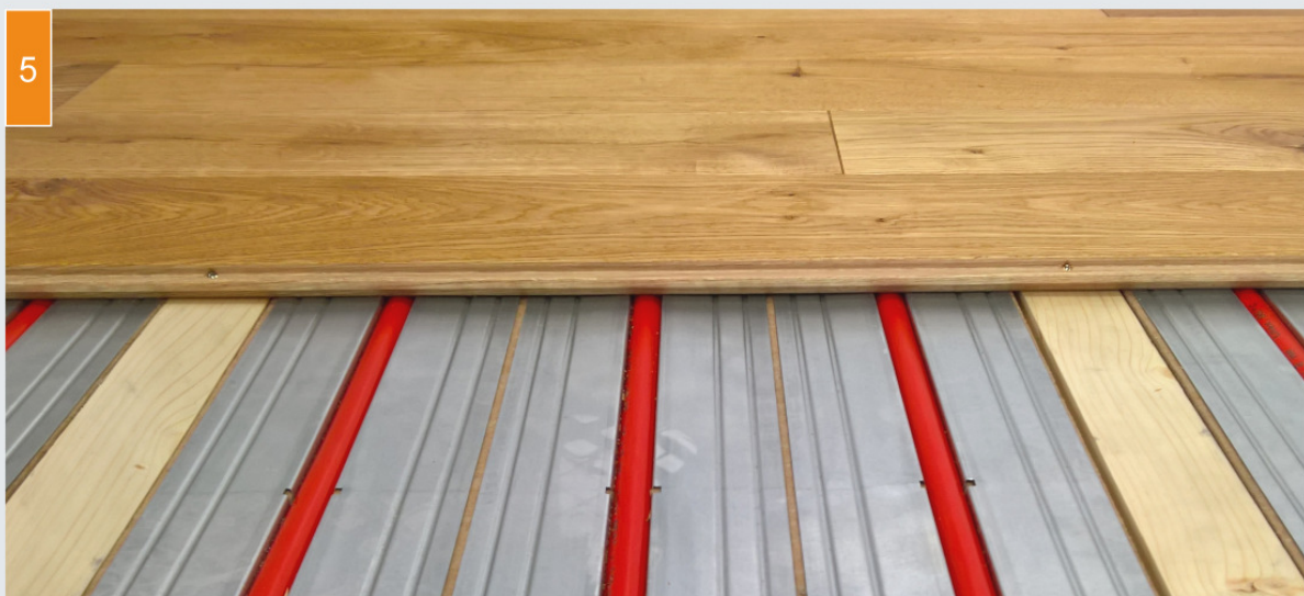
(5) A suitable wooden flooring is installed on top.
