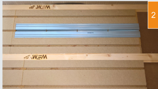
(2) Thermally conductive plates are laid in the fibre boards.
